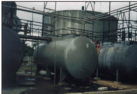
New tanks coated with ARC S4+ internally and ARC S2 externally
